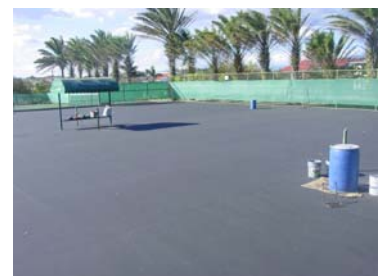
Application of the first layer on courts 7 and 8.
